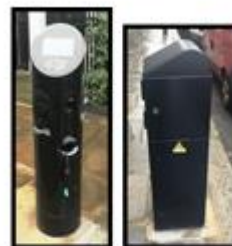
New Charge Point & Feeder Pillar
