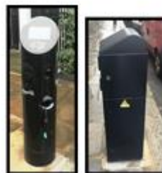
New Charge Point & Feeder Pillar
